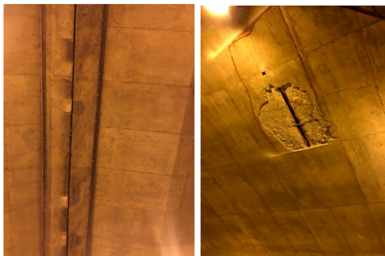
Figure 10: Dead End Anchor Corrosion, Strand Corrosion and Spalls at Lower Areas of the Bridge.
