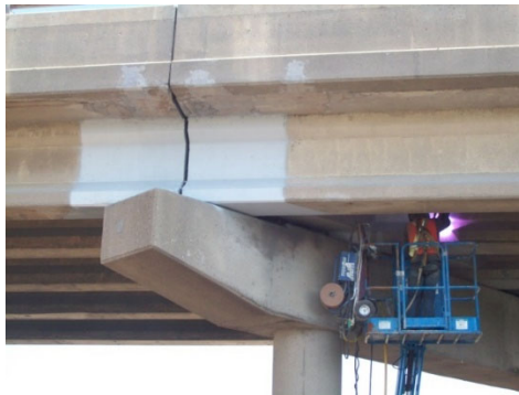
Figure 6: Galvanic Anode Installed to The Girder Ends to Mitigate Strand Corrosion
