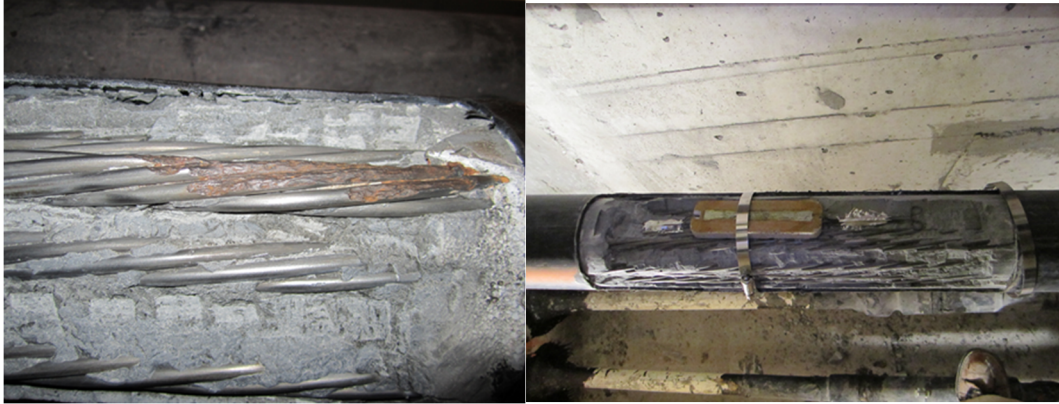
Figure 5: Galvanic Anode Installed to Mitigate Corrosion After Dissimilar Grout Accelerated Corrosion Discovered
