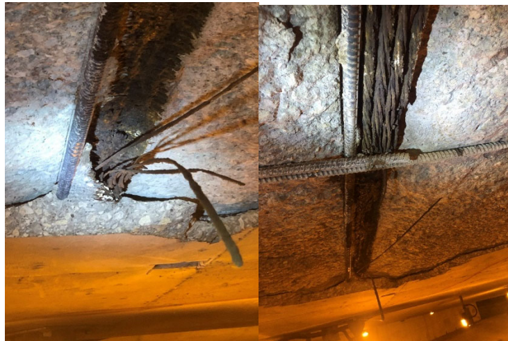
Figure 11: All 4 Strands Broken at Lower North Corner of the Soffit.
