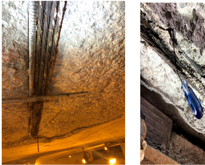
Figure 1: Prestressing Strands More Susceptible to Corrosion than Black Steel Regular Reinforcement - Strand Corrosion due to Poor Grout
