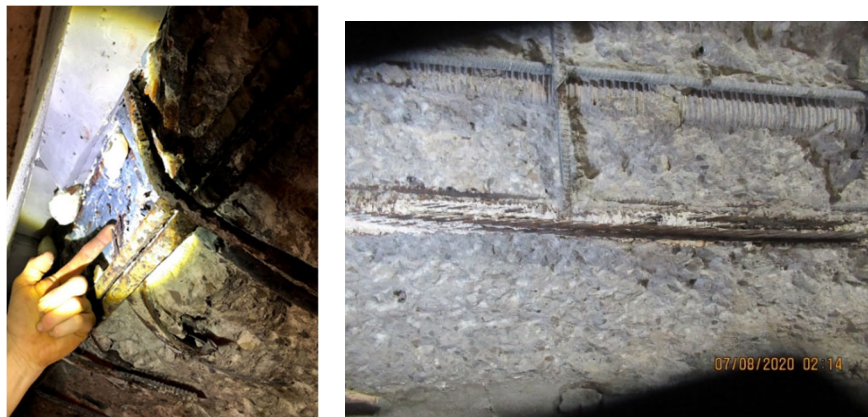
Figure 15: Dead End Anchor Corrosion, Strand Corrosion and Spalls
