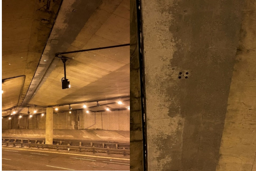
Figure 14: Activated Arc Sprayed Zinc anodes applied to the north soffit and connected to the steel
