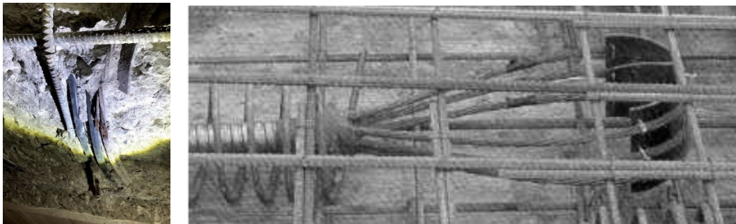
Figure 12: Looped Deadend Anchor Corrosion
